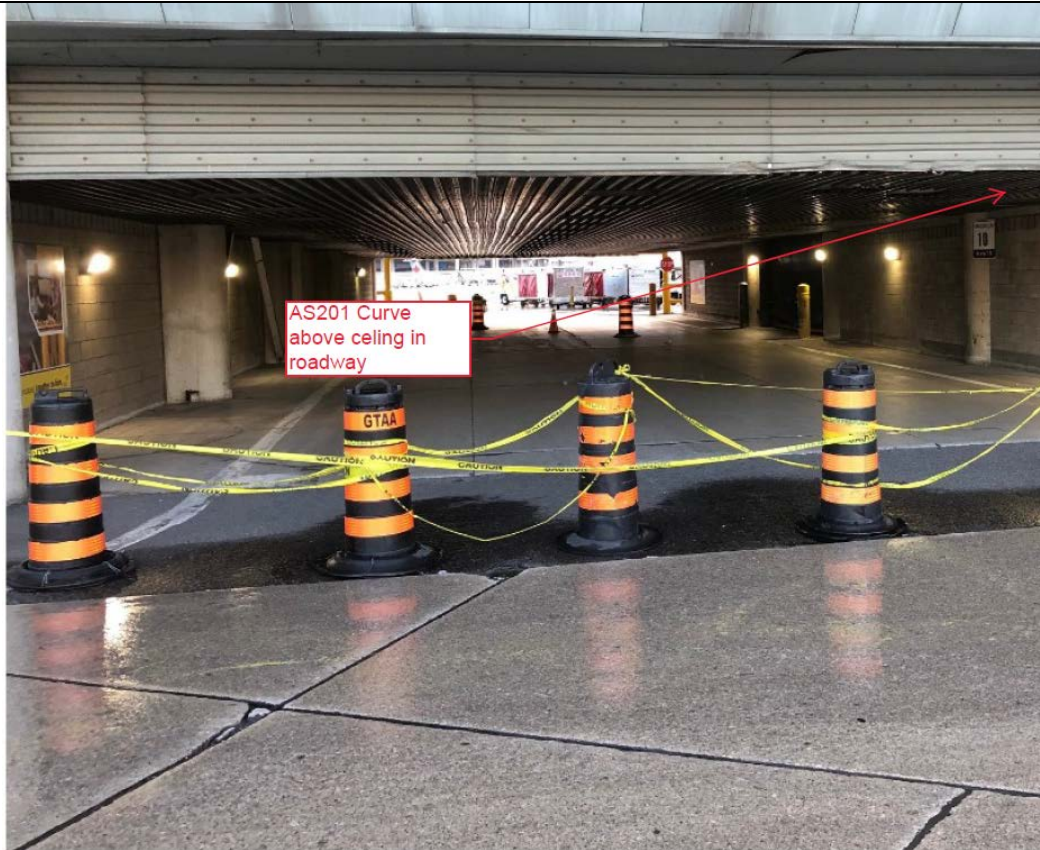
Figure 1 - Conveyor AS2-01 located above the ceiling of tunnel located near C27.
