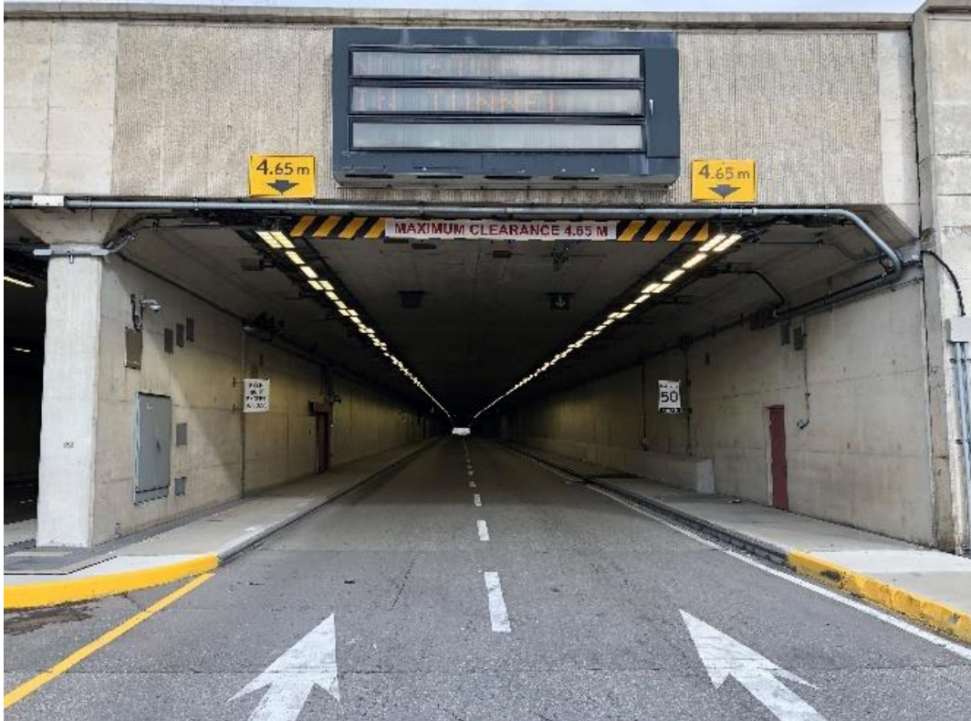
Figure 2-8: Infield Tunnel entrance to south cell.
