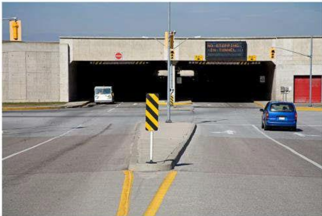
Figure 2-7: Entering the Infield Tunnel at the West portal.
