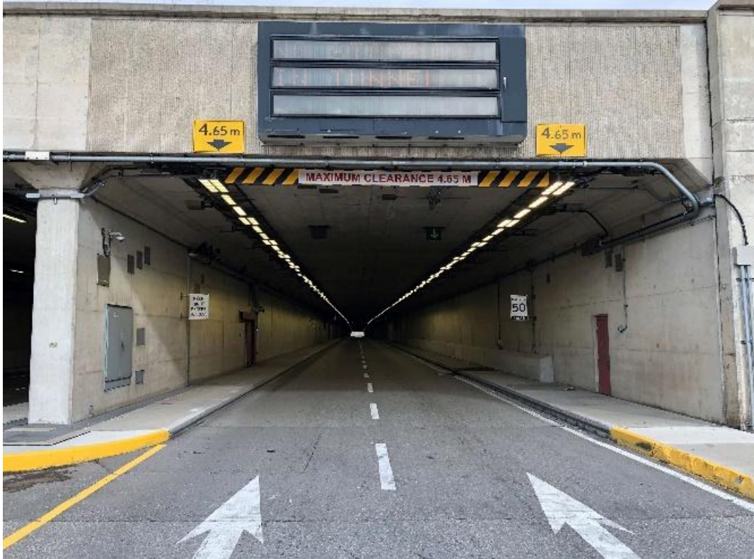
Figure 2-8: Infield Tunnel entrance to south cell.
