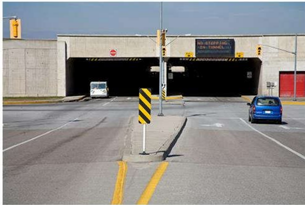
Entering the Infield Tunnel at the West portal.
