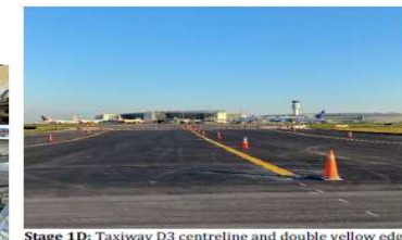
Stage 1D: Taxiway D3 centreline and double yellow edge markings painted.
