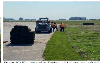
Stage 1C: Placing sod at Taxiway D1 along asphalt edge.
