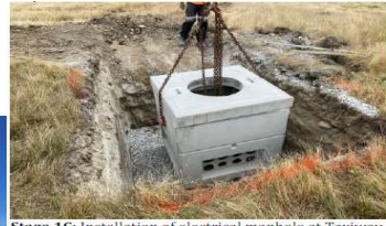
Stage 1C: Installation of electrical manhole at Taxiway stop bar.
