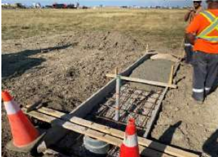
Stage 1D: Pouring the guidance signs base on Taxiway D3.
