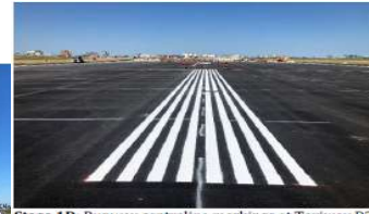
Stage 1D: Runway centreline markings at Taxiway D3 intersection (1 st coat)
