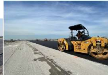
Stage 1C: Rolling and compaction of base asphalt on runway keel section.
