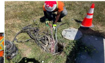
Stage 1C: Re-connect the cables from north runway side Taxiway D3 stop bar to the transformers in the pull pit
