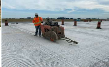
Stage 1C: Relief cuts on new PCC slab joints.
