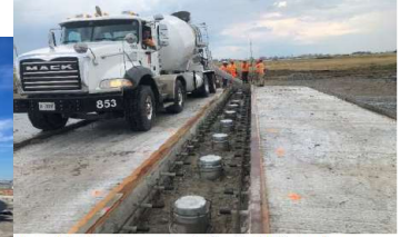
Stage 1C: Pouring concrete for Taxi D2 stop bar.
