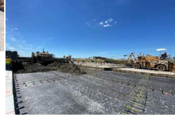
Stage 1C: PCC slip form paving via concrete belt feeder.
