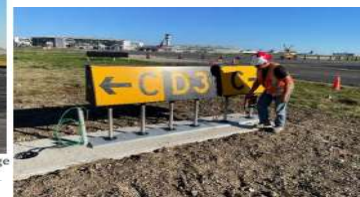
Stage 1D: Installing old D3 sign on new guidance sign base.
