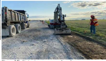
Stage 1D: Stripping runway edges for grass adjustments.
